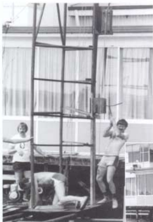
Driving the piles, 1982. For the new deck and the start of the renovations in 1983/84 for the Club House to what it is today
